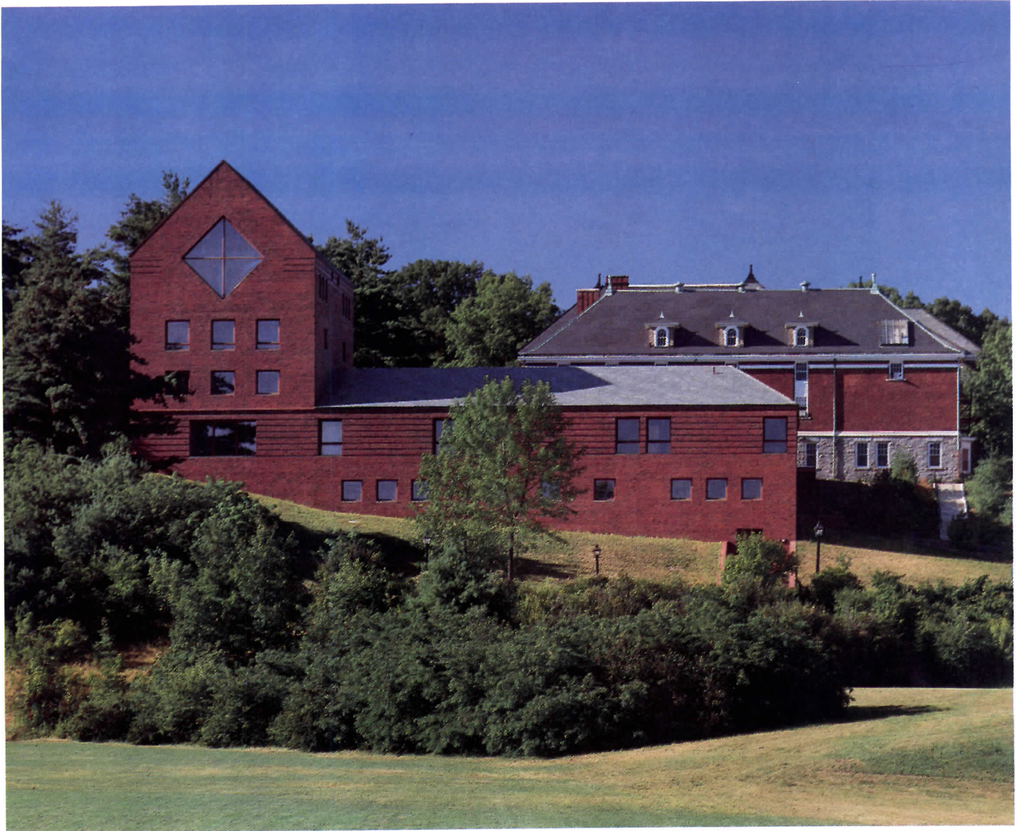
The dominant arch of the main entrance (opposite top) opens onto the main classroom floor from the quadrangle. The computer center is set into the slope below, with a secondary entrance at the far end (above). The horizontality of this block is emphasized by courses of green glazed brick. The three-story tower, with its big tipped-square window in the library, has a roof hipped in front, gabled at back.
