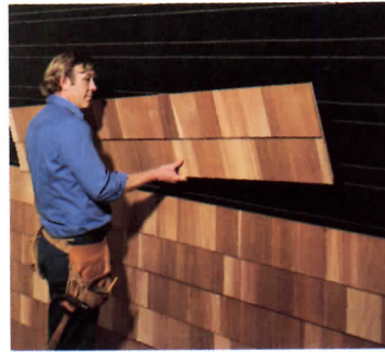
Put up 8-feet of shingles in a shake.
