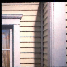
Faithfully detailed window moldings, trim and this extra-wide corner post.
