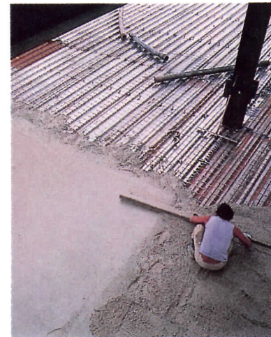
Composite deck simplifies construction
