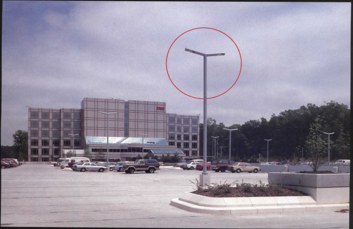
TRW Building, Fairfax County, Virginia
