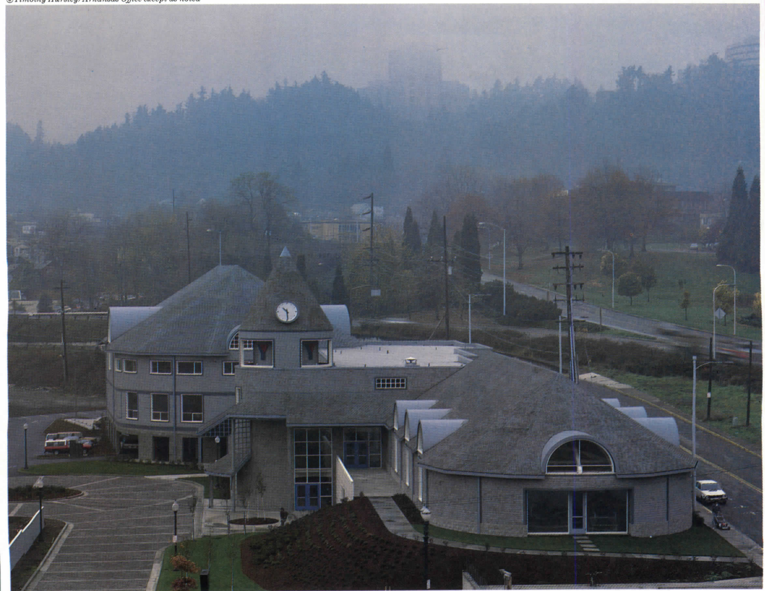
Separated from the skyscrapers of Portland's central business district by a major thoroughfare, RiverPlace sits on the banks of the Willamette River like a quiet Pacific Northwest village (opposite top). Anchoring the north end of its 10-acre site is the athletic club designed by the Zimmer Gunsul Frasca Partnership. In evoking the proportions of a Richardsonian building, the new facility has become an instant landmark for the new waterfront community.
