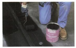
Coating both cleaned membrane splice-widths with EP-95 Splicing Cement.
