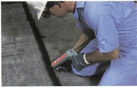
Applying Lap Sealant to the splice edge.
