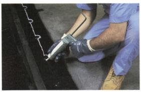
Applying In-Seam Sealant according to specifications.
