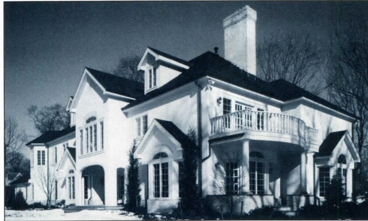
A house very closely resembling this one designed by architects Nadler, Philopena & Associates was built last year only a few doors away from the original
