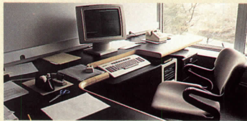
Installed at desktop level, the Wiremold perimeter raceway in this office handles both standard power and low voltage communications wiring.
