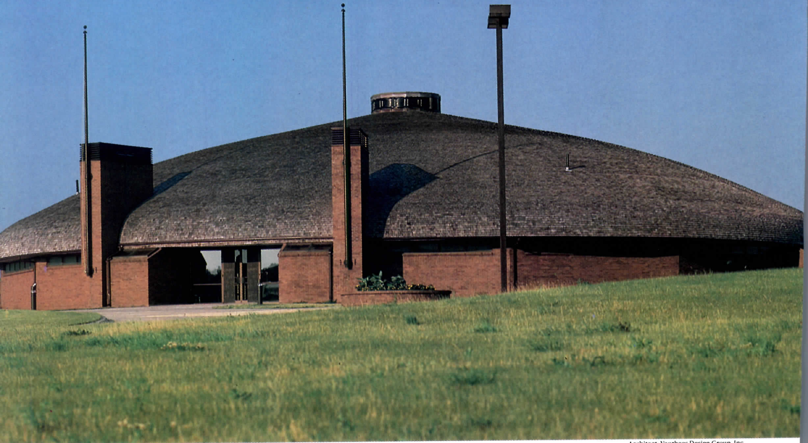
Architect: Voorhees Design Group, Inc.
