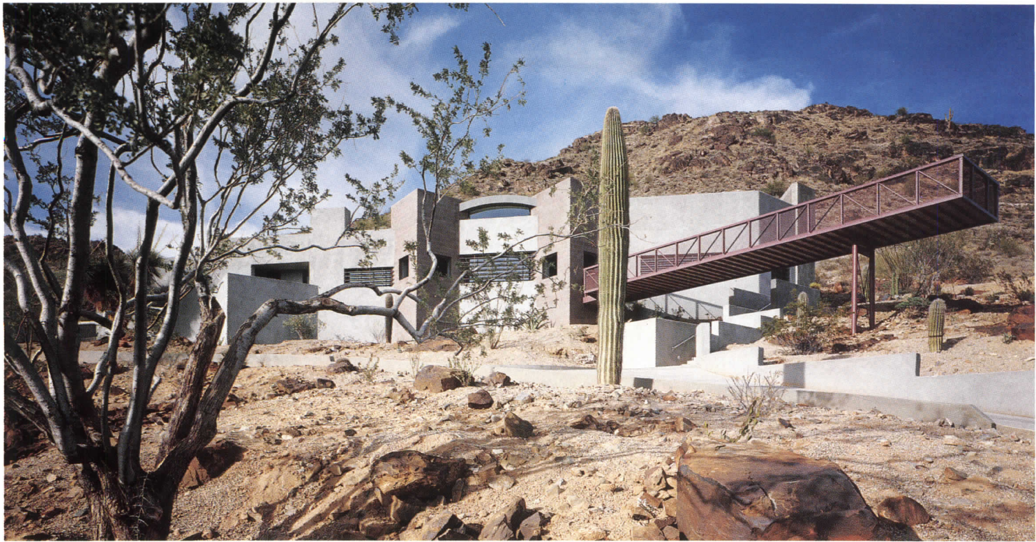
A steel bridge, both entrance gateway and terrace, addresses the displaced-land allowance dictated by town code.
