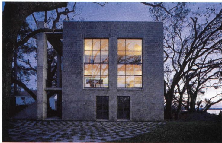
The north facade features 17-foot-tall industrial windows.
