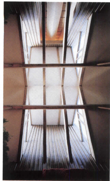
Clerestories (top left and above) formed where structural members intersect bathe studios with light. A custom four-foot square pendant hangs above the client's studio worktable amid a forest of exposed columns, beams, and braces (bottom left and opposite).
