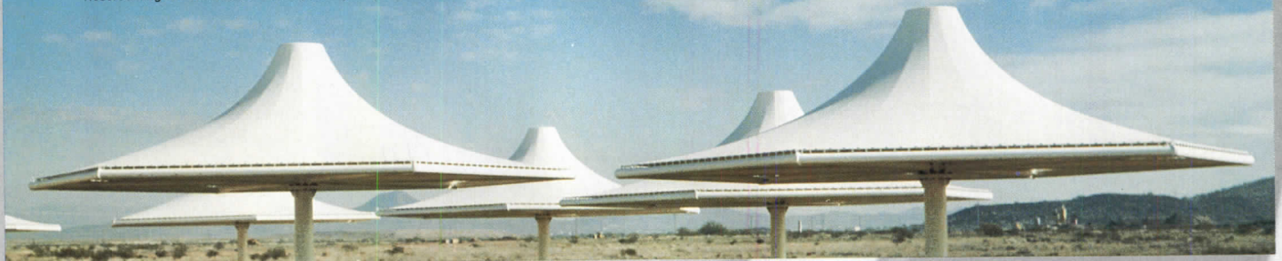
Individual Modular Shelters, Phoenix, Arizona.
