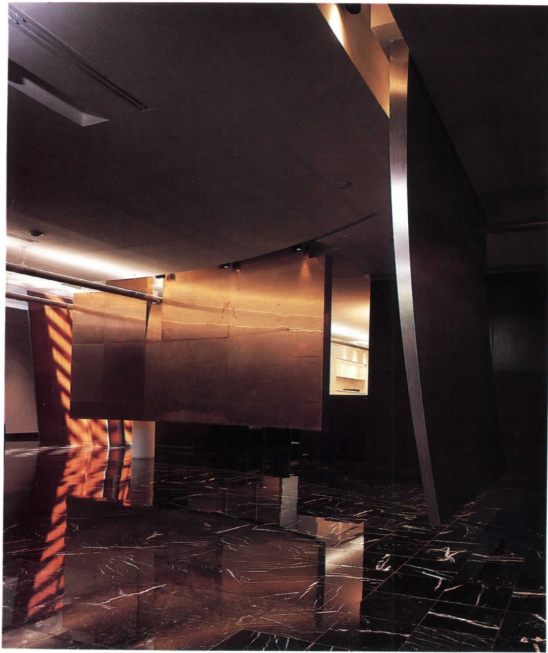
Curved metal partitions hang from the ceiling.
