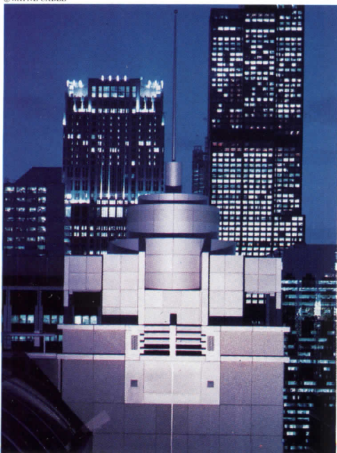
One of two pairs of painted-aluminum spires atop 225 West Wacker Drive, in Chicago.
