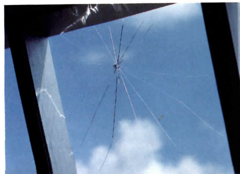
If a flying object damages only an outer light, a laminated-glass pane will usually remain within its frame.
