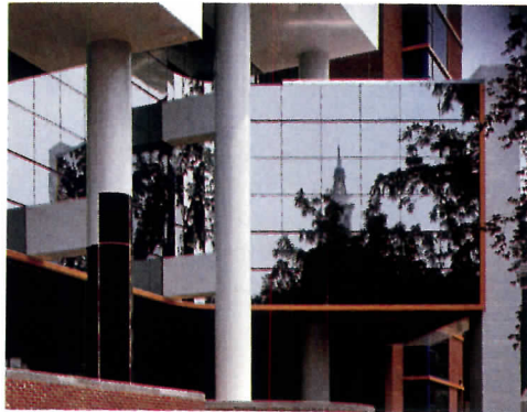
Curtainwall using Duratec glass; Sherman/Carter/Barnhart, Architects.
