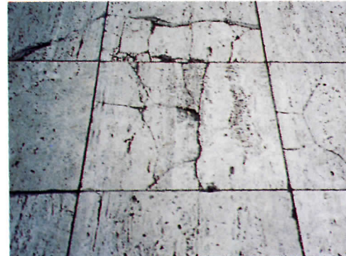
Stone damaged by differential movements: at a connection (top left), above a window (bottom left), and pavement over a structural slab (above).
