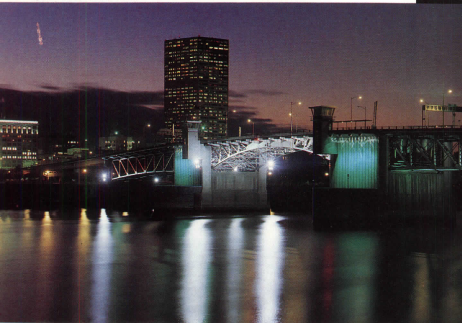
Four floodlights mounted on the piers play on the rugged structure of the Morrison Bridge . Color comes from plastic gels on the luminaires, which are changed periodically.
