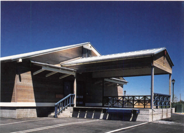
The post office's stepped false-front facade (top) mimics the most distinctive feature of turn-of-the-century Western architecture, and its enclosed outdoor bench was modeled after a former stop on the old Butterfield
