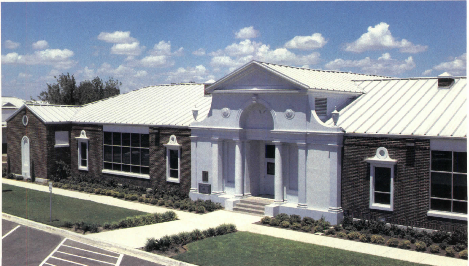
Project: Sharyland I.S.D. Administration Building Renovation Architect: Boultinghouse, Bustos & Associates Roofing Contractor: Bullard Sheet Metal & Roofing Co. Roofing Material: MBCI's Standing Seam Ultra-Dek 124® , Bare Galvalume
