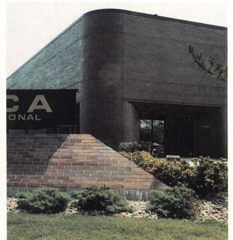
Building Officials & Code Administrators International, Inc., Flossmoor, Illinois Architect: Linden Group, Inc. Photo: Linden Group, Inc.
