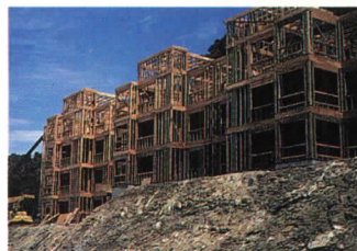
Wood frame structures are cost-effective in high density areas and difficult terrain.
