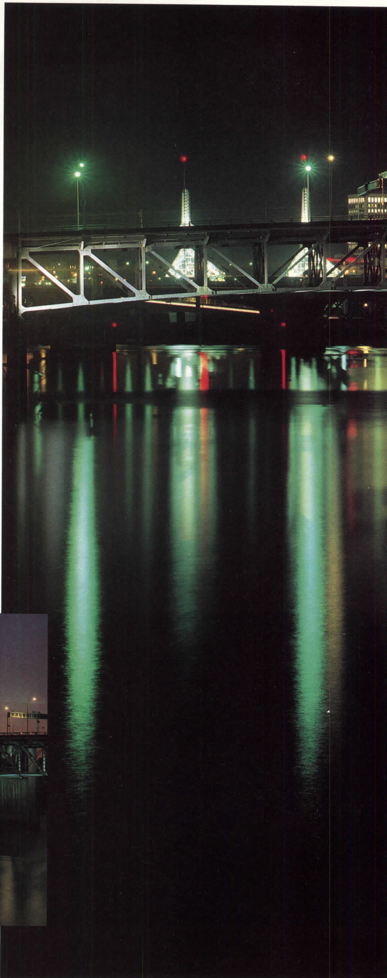
Four floodlights mounted on the piers play on the rugged structure of the Morrison Bridge . Color comes from plastic gels on the luminaires, which are changed periodically.
