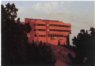
Award of Excellence for multi-story wood design by Shen/Glass Architects, Berkeley, CA.
