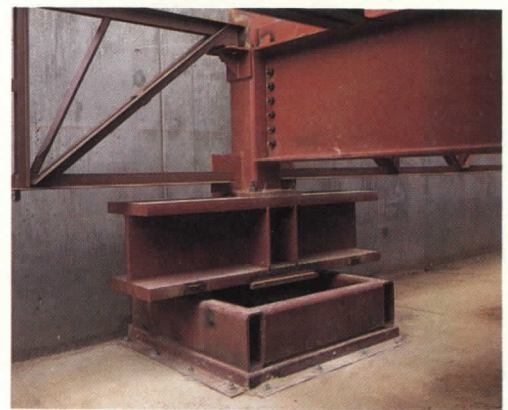
The design team chose a "base isolation" system to accommodate seismic loads. They also specified Vulcraft steel joists and joist girders for the building.
