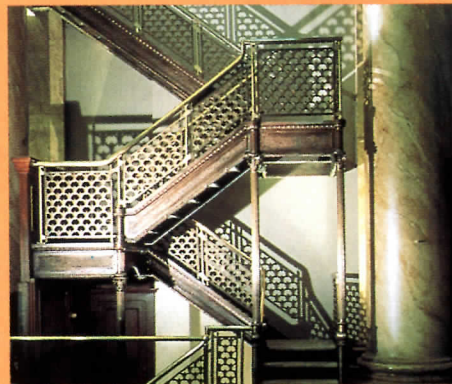
Left: The monumental-stair problem as shown in the New York State Capitol before remodeling by The Ehrenkrantz Group. Right, top: The open fire-stair problem in The Bowery Savings Bank,
