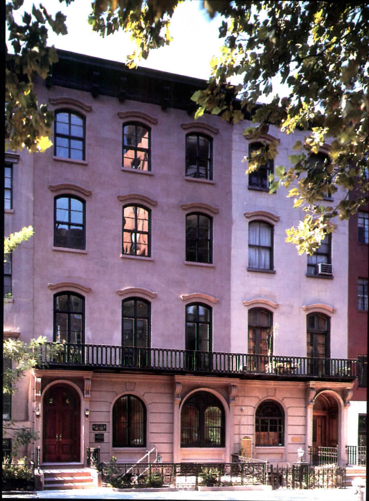
Casa Italiana Zerilli-Marimò New York University New York City Helpern Architects
