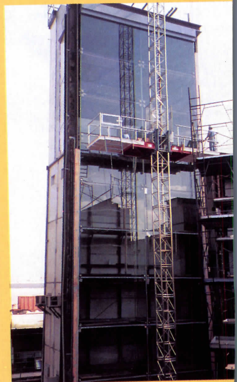
Testing of a 21-by-64 foot all-glass curtain-wall mockup at the Construction Research Laboratory.
