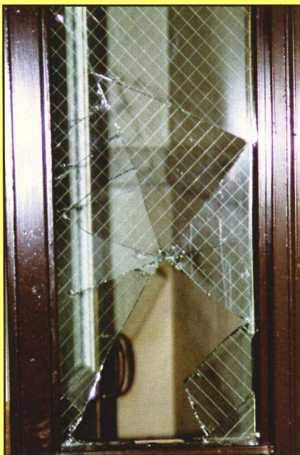
Wired glass prior to removal
