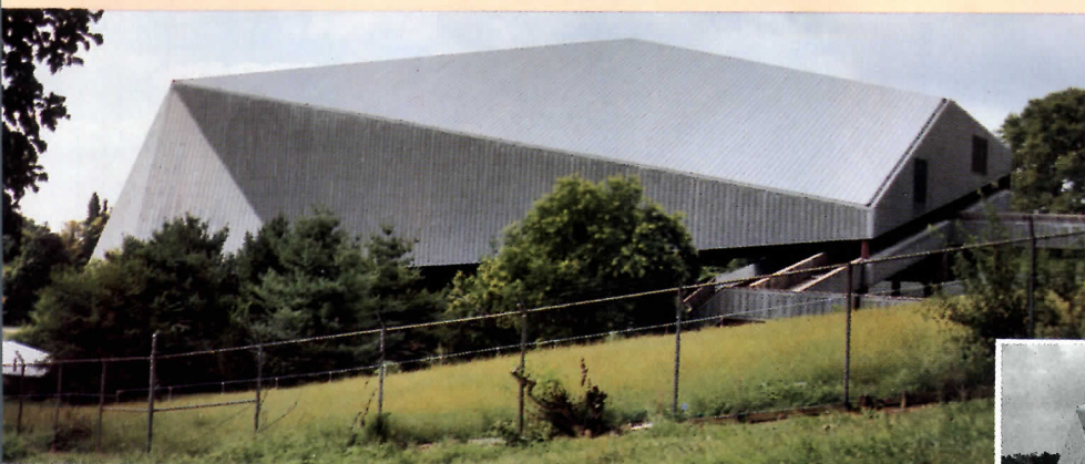
Robin Hood Dell, Fairmont Park, Philadelphia, PA. More than 50,000 square feet of TCS roofing shown after 16 years of weathering.
