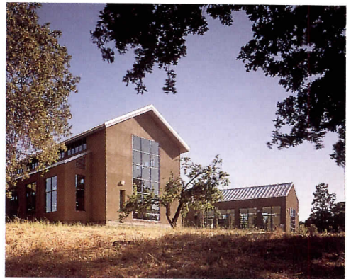
The $2.8-million library is a simple steel-frame structure clad in colored stucco that picks up the hues of the surrounding landscape. Although the architects had explored several roof options, the community expressed a strong desire for a gable design that recalls agricultural buildings.
