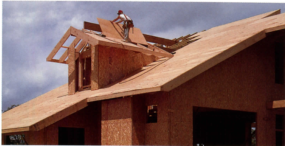
APA trademarked engineered wood products are used in residential construction on floors, walls and roofs.
