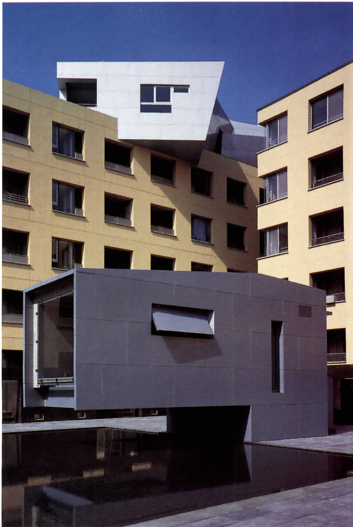
A view from inside the “Water Reflecting House” (opposite). It cantilevers over a pool (below left).
