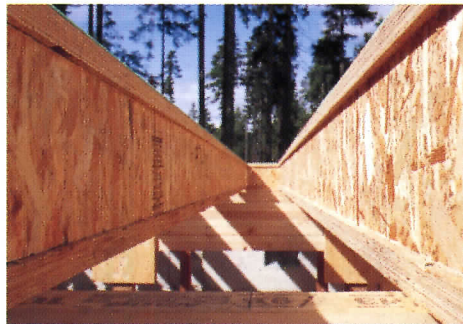
APA EWS trademarked engineered wood I-joists allow you to use longer spans and wider spacings than standard lumber joists
