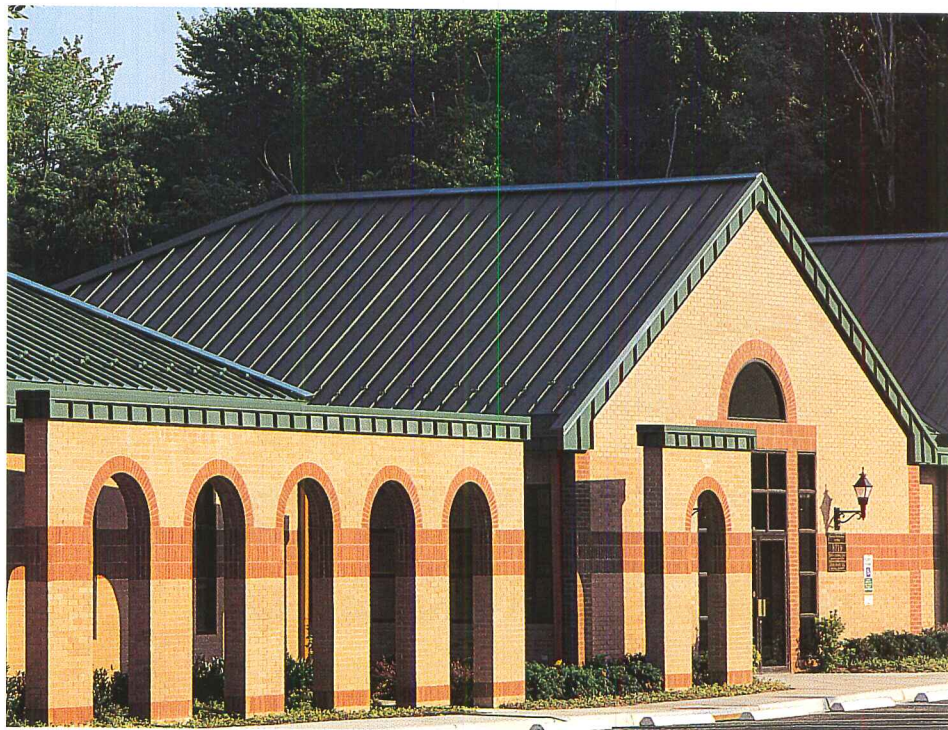
Dental Offices of Manassas Architect: Robert Loveless General Contractor: Rector Construction Roofing Contractor: GRC Roofing Inc. Color: Forest Green Profile: 24 ga. SNAP-CLAD
