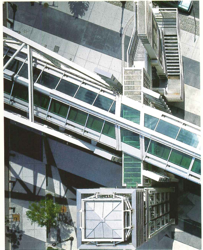
Tribeca Bridge, Skidmore, Owings & Merrill
