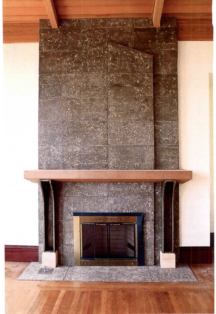
Craftsman Buddy Rhodes colored this chimney piece with liquid pigments, and cast the concrete with a random-vein pattern.
