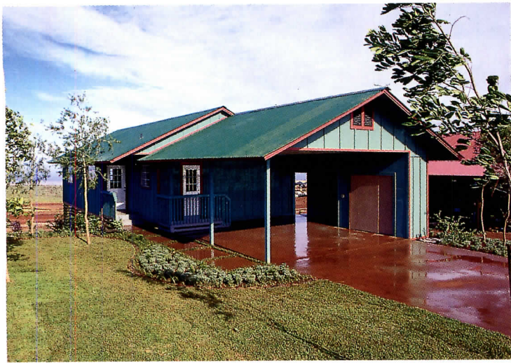
A low-budget use of colored concrete: the drive and walkway of a Hawaiian bungalow are tinted to blend with the red volcanic soil.
