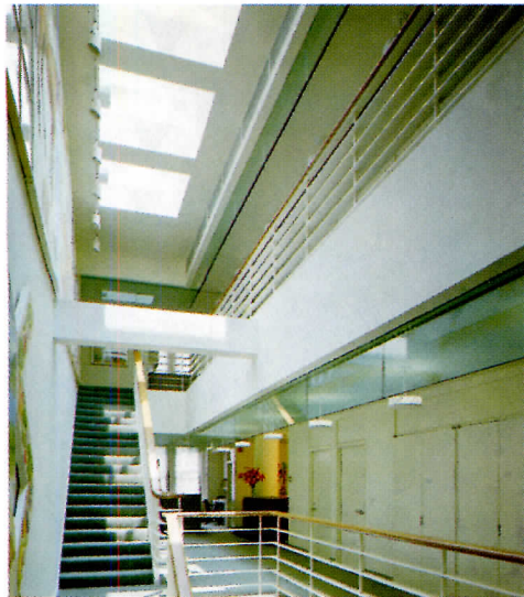
At the NRDC Building, the Croxton Collaborative brought daylight in from a skylit atrium (left). At Audubon House, the firm used glass partitions to allow sunlight to penetrate deep into the offices (below).
