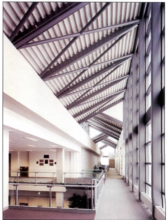
Photo: MacAlester College, St. Paul, MN Architect: Holabird & Root Photo By: Steven Bergerson Photography, Minneapolis A/D FIREFILM® on structural steel
