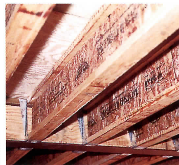
The Bass Lofts at Atlanta's Little Five Points is one of the first multi-unit housing projects to include Georgia-Pacific's newly standardized wood I-joists. The project, shown here in various building stages, includes the conversion of a school into lofts and a new apartment building.
