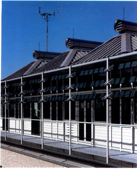
Glass louvers shade the windows and reduce glare (left). The six-inch-deep floor plenum (right) contains a central spine of data and power cabling. Heat, air-supply, and white noise controls at each workstation plug into this spine and the adjacent ductwork.
