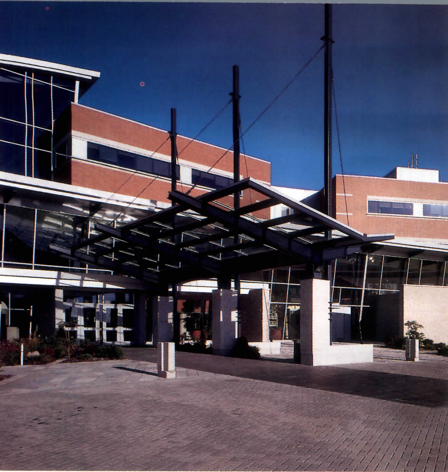
The main entrance to the headquarters is marked by a metal-and-glass canopy (above). Public elements such as the library (right, top and
