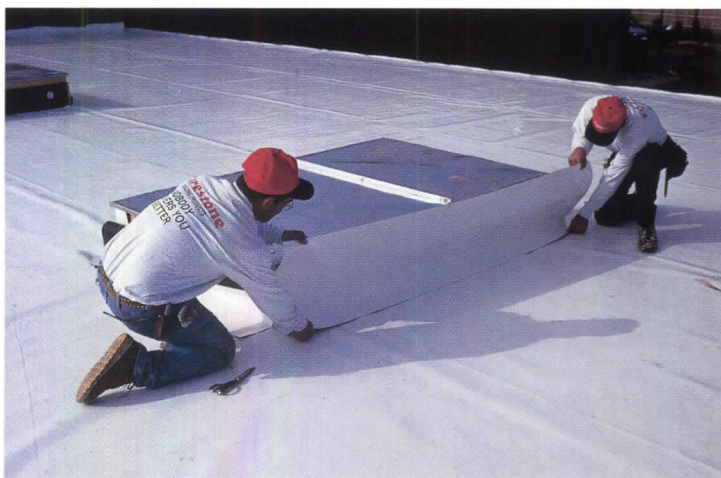
Narrow rolls of TPO are labor intensive to install, but are more stable.
