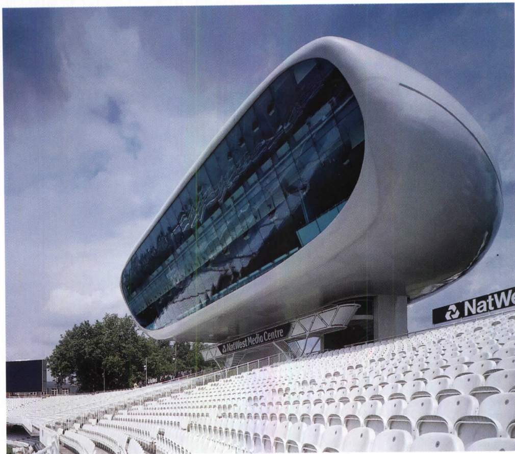
The media center had to be prefabricated in shipyards and cost over $9 million to construct and install.
