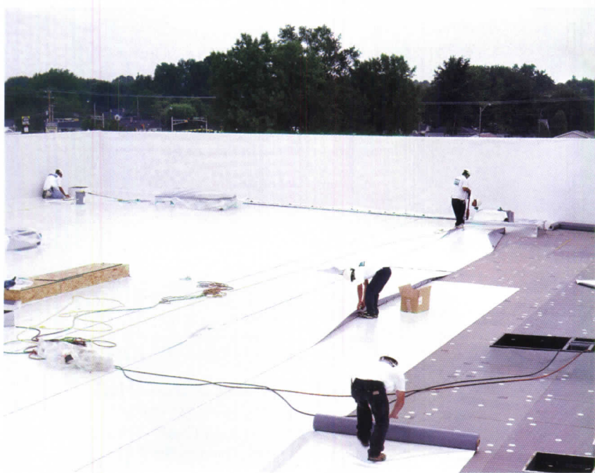
Heat-welded PVC seams are stronger than the membrane in the roof field.
