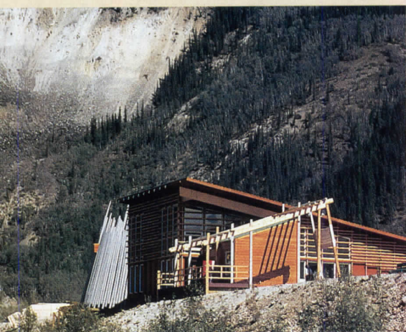
Located in a remote area of the Yukon, the Tr’ondek Hwech’in Cultural Centre by Maurer Kobayashi Architects (opposite top right and above) is a tribute to the Han people. Because the structure itself incorporates references to various built forms the Han used, such as their fish-drying frames, skin-and-stick tents, and basket traps, the building itself is a museum to the people.
