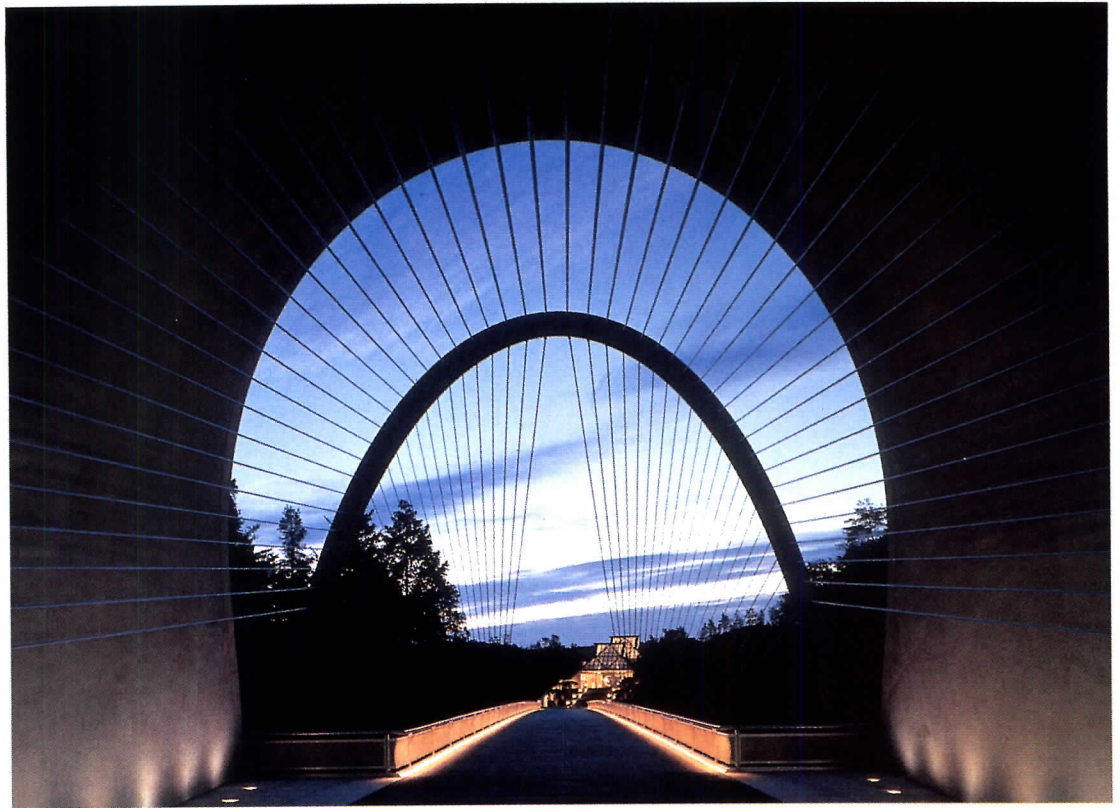
The 44 cables resemble a parting veil as pedestrians pass from the tunnel to the bridge (above). The posttensioned cables fan out (right) after passing through threaded rods in the arch (far right) and are anchored to the space frame.
