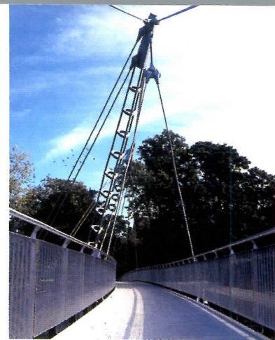
The slender cable-stay bridge at Maidstone (left) spans both a river and its floodplain. The cables are strung from two lacy masts (above).
