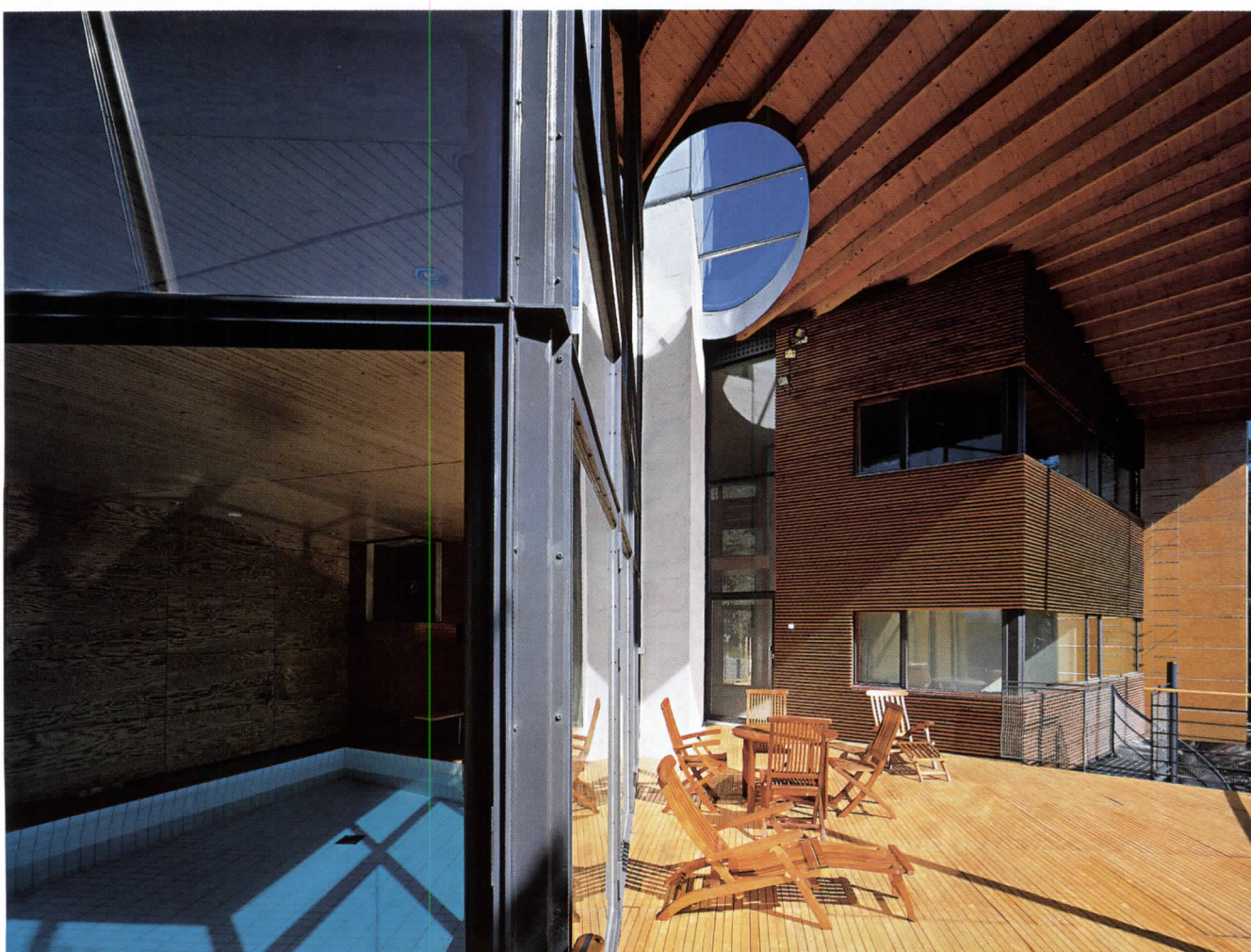
Skewed steel columns, cable-stayed and footed directly to the granite, accentuate the project's language of tension and suspension (opposite). With various types of wood, including cherry floor boards and pine-veneer plywood wall panels in the living room (this page top), Tasa creates a range of textures. The pendant living room lamp is of his design. A deep deck (this page bottom) extends the glass-enclosed swimming area to the outdoors.
