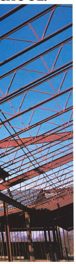
Take a lesson from the Bransford Elementary School in Grapevine, Texas. Where the structural engineer saved money using Vulcraft sloped seat steel joists instead of wood construction
