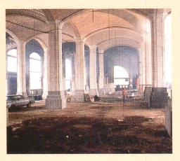
toward the river, while the roof, supporting the roadways above, slopes up from the city streets to the bridge's river-crossing segment. The vaults contain four layers of backing tile and one layer of so-called face tile; each vault contains more than 1,600 face tiles.
