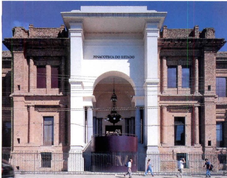
Exterior of State Pinoteca, with interventions such as removed window frames.
