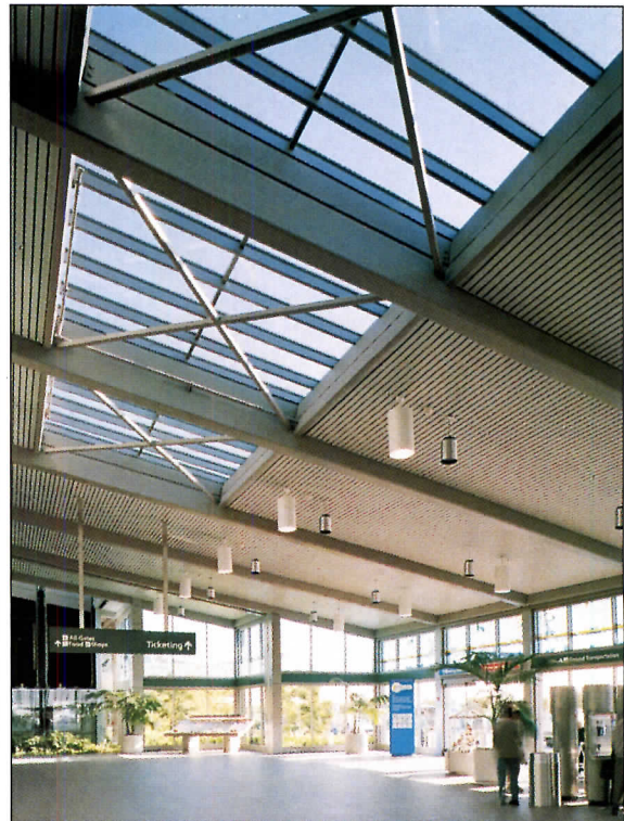
Photo: Sacramento International Airport, Terminal A Architect: Dreyfuss & Blackford Architects Photo: Cathy Kelly Architectural Photography A/D FIREFILM® II on structural steel.
