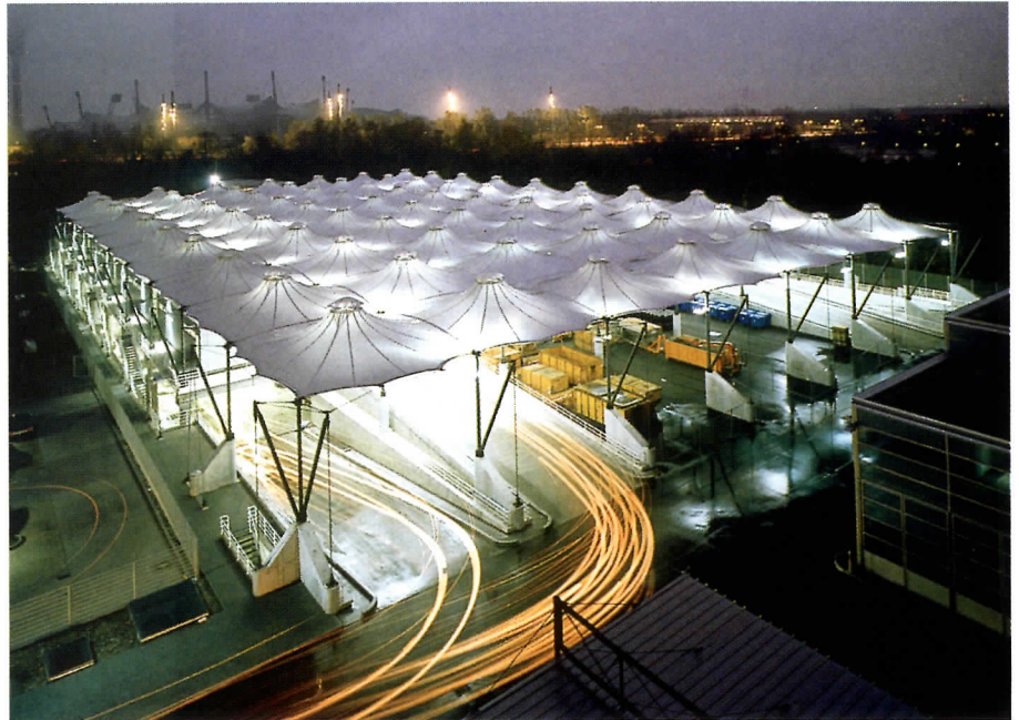
The AFA Carport in Munich illustrates one of the main advantages of fabric—large areas can be covered using a minimal amount of structural material.
