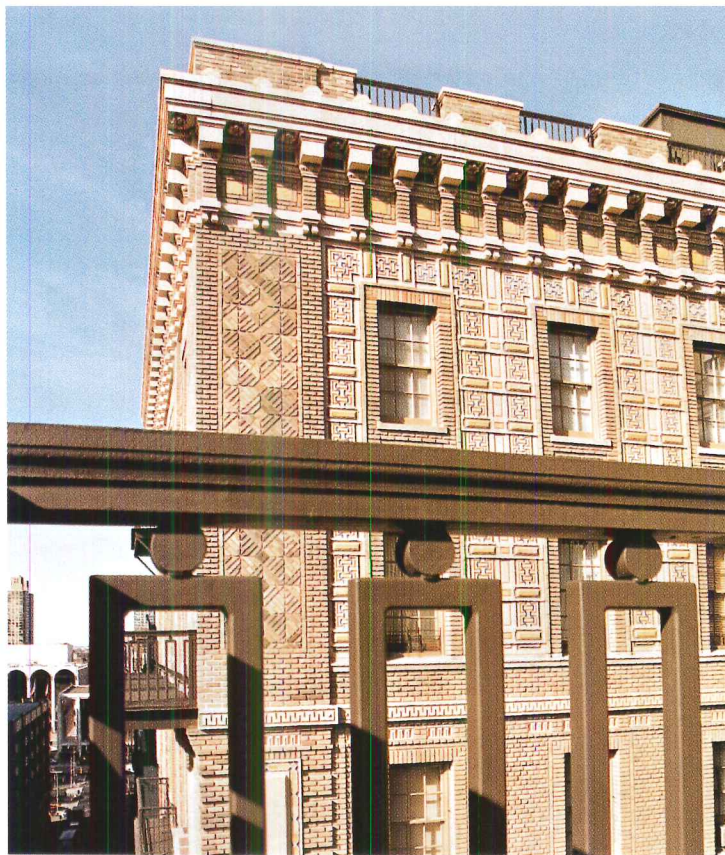
The balconies were removed, refurbished, and the steel structure replaced.
