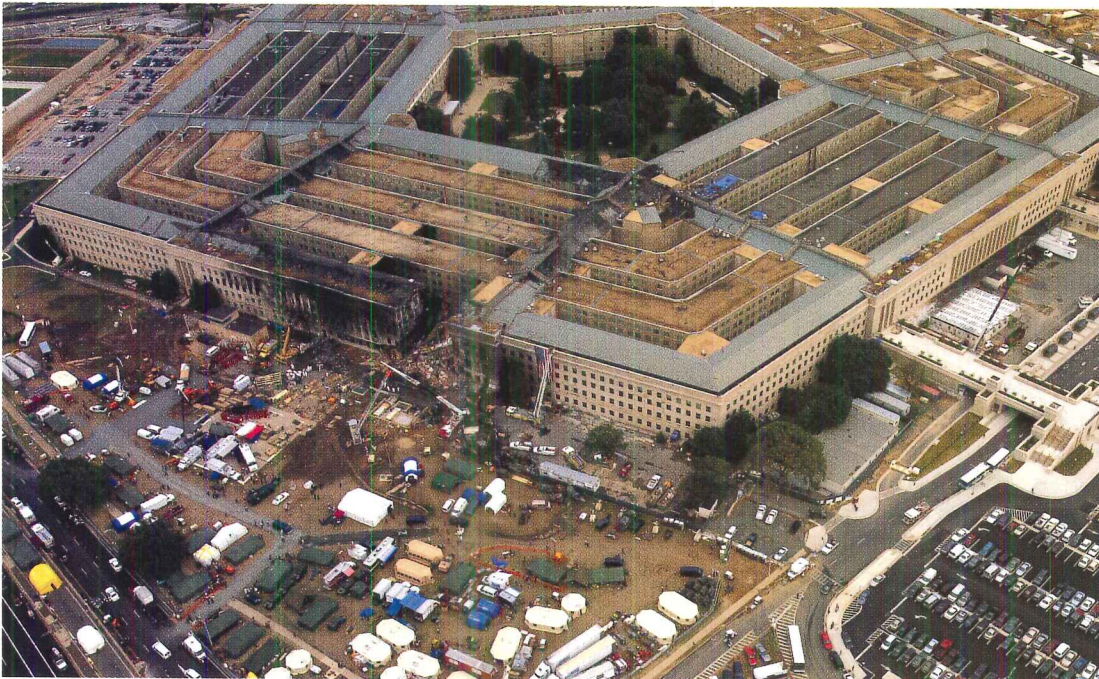
While a relatively small portion of the Pentagon was destroyed on September 11, the estimate to rebuild is $520 million.
