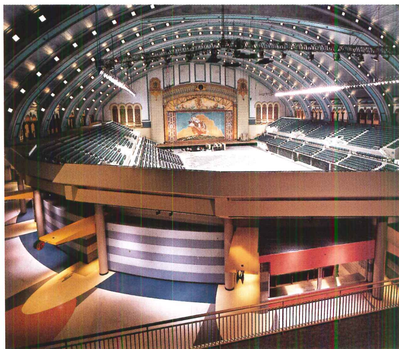
A new precast seating bowl improves sight lines, capacity, and comfort.
