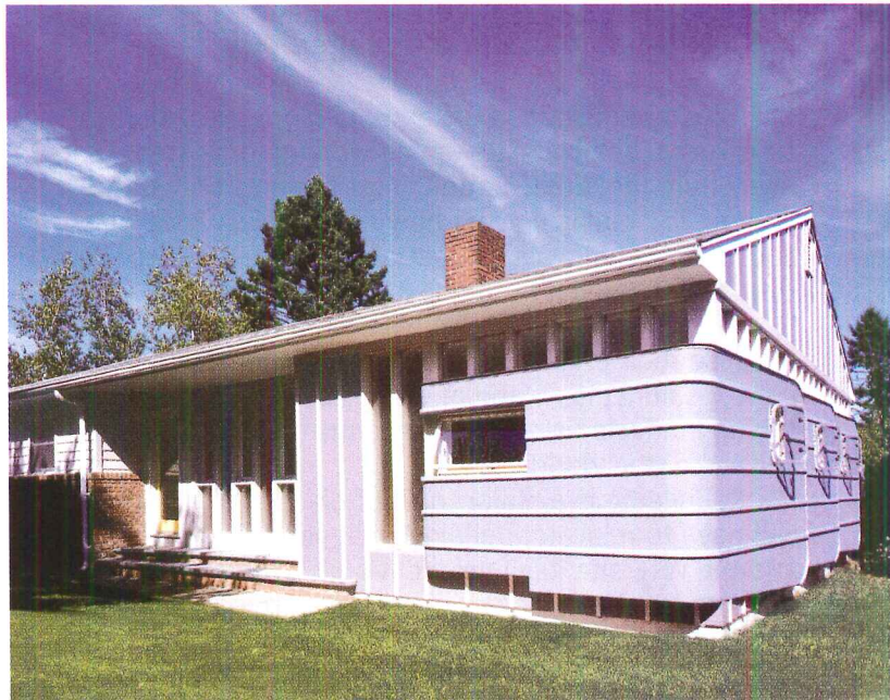
Ranch House Addition, Amagansett, NY, 2001
