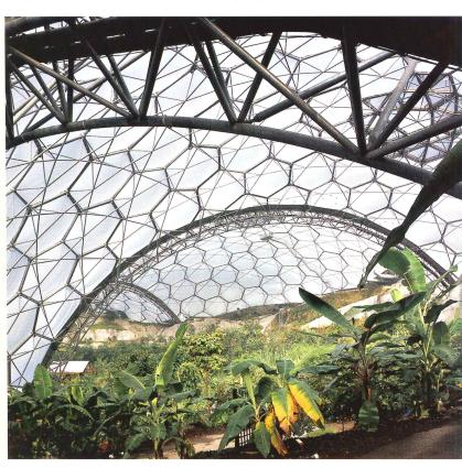
Mero, a space-frame fabricator, suggested adding a layer of triangulated struts under the hexagonal panel's chords (temperate biome, opposite). This eased construction because the panels could be erected in sections and remain self-supporting. Unit heaters augment natural ventilation (below). Inside the tropical biome (bottom).
