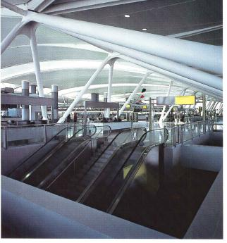
Skylights in the roof (far left) reinforce major lines of circulation. The food court, one flight below the departures level, is open to the bowed, unifying roof (left). The truss, formed by a series of tripod supports, meets the roof with moveable joints that flex with snow and wind loads.
