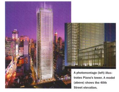
screens 18 inches from one skin of transparent glass will be a second skin with about 250,000 white ceramic rods, 1% inches in diameter. The rods will filter sunlight but will be spaced to allow views outside. The building itself will be 748 feet tall, but the ceramic screens will reach 840 feet, and a central mast will top out at
