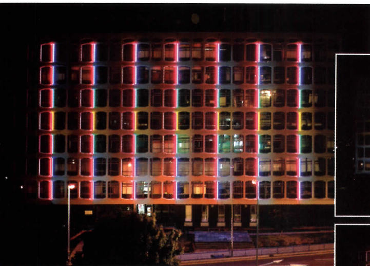
The facade lighting project incorporates 86 individually controlled, 10-foot-long cold-cathode tubes.
