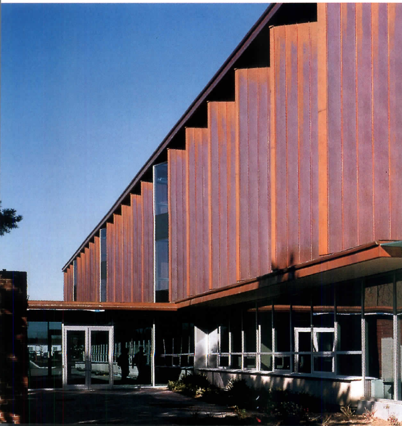
The copper-clad facade with a sawtooth pattern on the building's east and west sides (west side shown here) allows for winter solar gain and summer shade on the east; it is oriented for northern light on the west.
