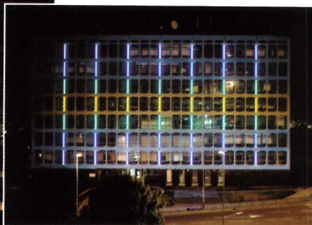
The facade lighting project incorporates 86 individually controlled, 10-foot-long cold-cathode tubes.
