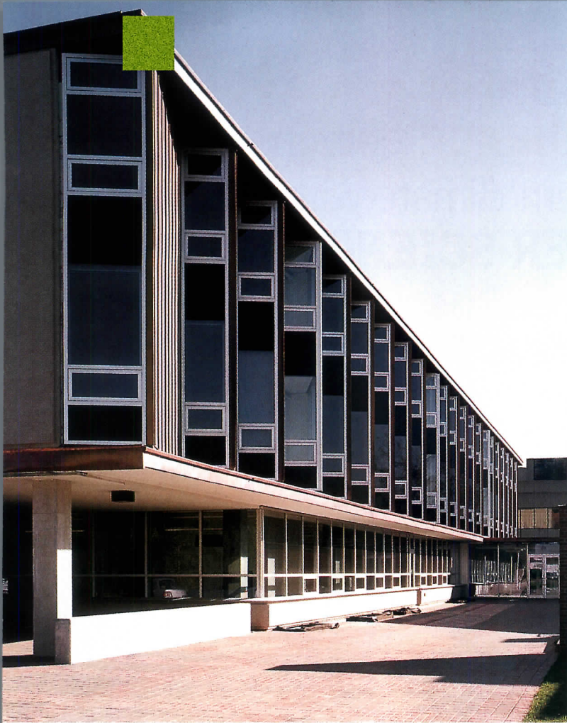
The copper-clad facade with a sawtooth pattern on the building's east and west sides (west side shown here) allows for winter solar gain and summer shade on the east; it is oriented for northern light on the west.
