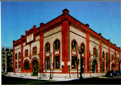
Renovated in 2001 by Holst Architecture, the Jean Vollum Natural Capital Center in Portland, Ore. (left), is the first historic building to receive a LEED gold rating.
