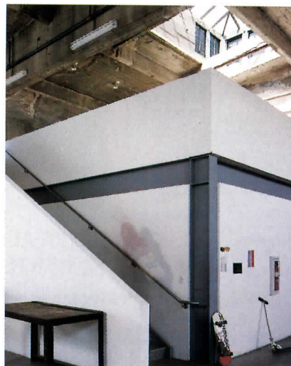
The strong points of the library (far left) are its high ceiling and abundant natural light. Steel mezzanines (near left and below) increased the building's floor space by more than 50 percent.
