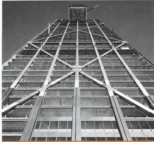
1970 Cross-bracing is an innovative exoskeleton for the tube structure of Chicago's John Hancock building. The x-shaped bracing creates strength while saving material.
