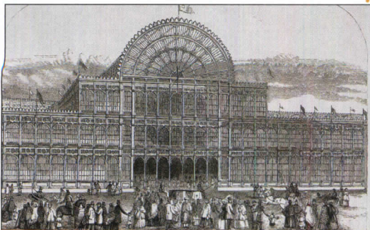
1851 London's Crystal Palace is an example of one of the first buildings made of prefabricated cast-iron parts.
