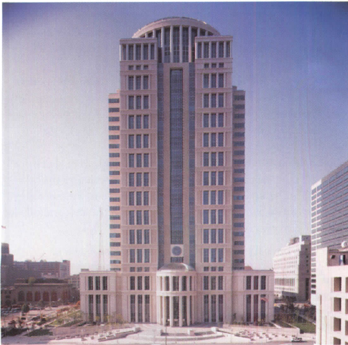
The Eagleton Center, a Federal building in St. Louis, Missouri, is a 27-story structure of precast panels colored with CHROMIX Admixtures in a custom color that also matches the surrounding hardscape.
