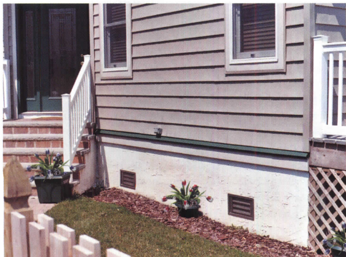
Smart VENT® Installation
