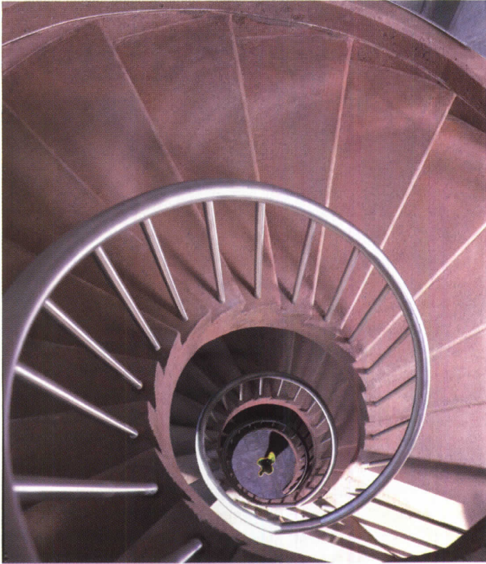
This stunning free-standing spiral staircase rises four stories in Montvale, a private home near Atlanta. Integrally colored with CHROMIX Admixtures Dusty Mauve.
