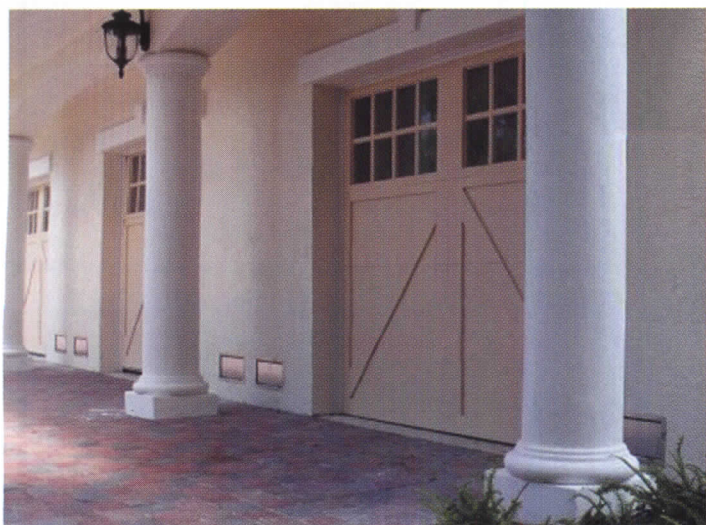
Flood VENT™ Installation
