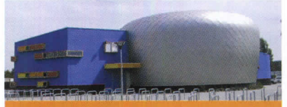
1990s Titanium, rust-free and corrosion-resistant, makes an architectural statement on buildings around the world.
