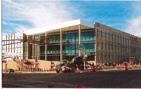
Finishing up the new federal building.
