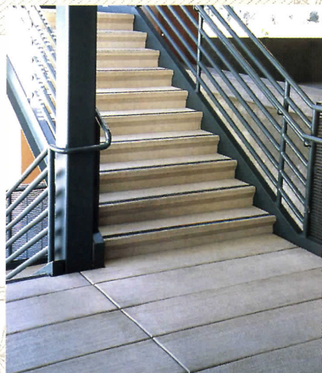
PRECAST CONCRETE CLOSED RISER STAIRTREADS AND LANDINGS. ADA COMPLIANT
