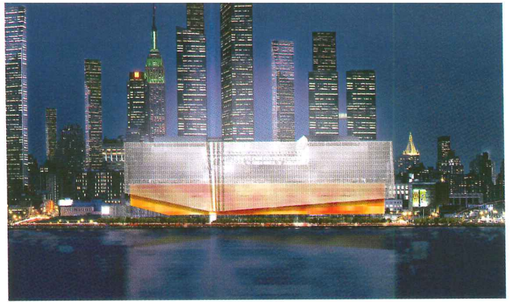
The new design for the stadium is draped by a glass “veil” (above) with an LCD screen on its lower levels.
