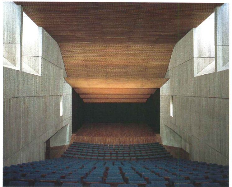
Throughout the interior, the architect played accents of tropical iroko against exposed board-formed concrete—as seen in the auditorium (below) and lobby (opposite). A steel stair (above) rises from the back of the foyer to a café with an outdoor terrace.
