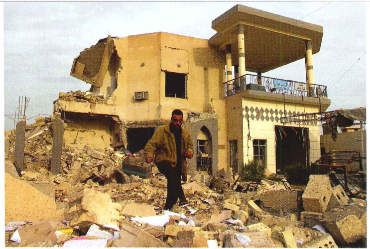
Although many buildings were destroyed during the Iraq War (above, a civic structure in Ramadi), looters are responsible for the most significant losses.
