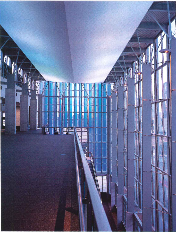
The blue-glass screen shading the west elevation is visible beyond the balcony (above). Skylights over wedge-
