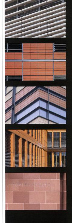
Façade design with large-format ceramic elements for a unique architectural style.
