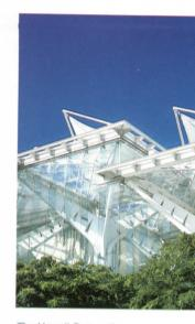
The Hawaii Convention Center, Architect: Wimberly Allison Tong & Goo. Design and Planning: LMN Architects. Features the largest suspended glass wall in the U.S. fabricated by Oldcastle Glass® in Stackwall."
