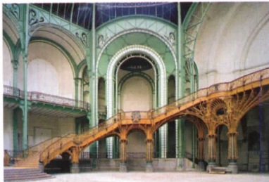
Bright, elegant Grand Palais renovation.
