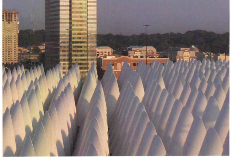
For the new museum restaurant (left), the Woodruff Arts Center commissioned an illuminated artwork by Spencer Finch. Light scoops atop the new gallery roofs (above) filter northern light into loftlike galleries. Additional skylights (right) can be temporarily masked to adjust daylight levels.
