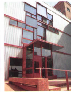
Higgins Hall's center section, by Holl.
