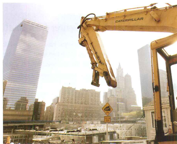
Freedom Tower construction under way in April.
