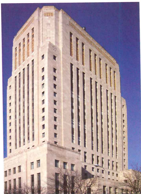
The 1934 Jackson County Courthouse recently underwent a complete exterior renovation.
