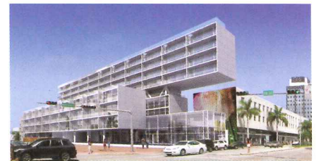
The building will have a 54-foot-long cantilever.
