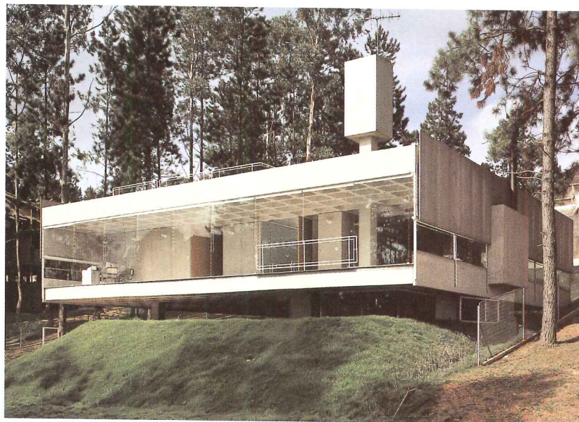
Una Arquitetos' FDE Public School (top) replaced an ineffective facility with a luminous, open-feeling one. MMBB's Mariante House (above) employs concrete as a delicate, non-load-bearing element.
