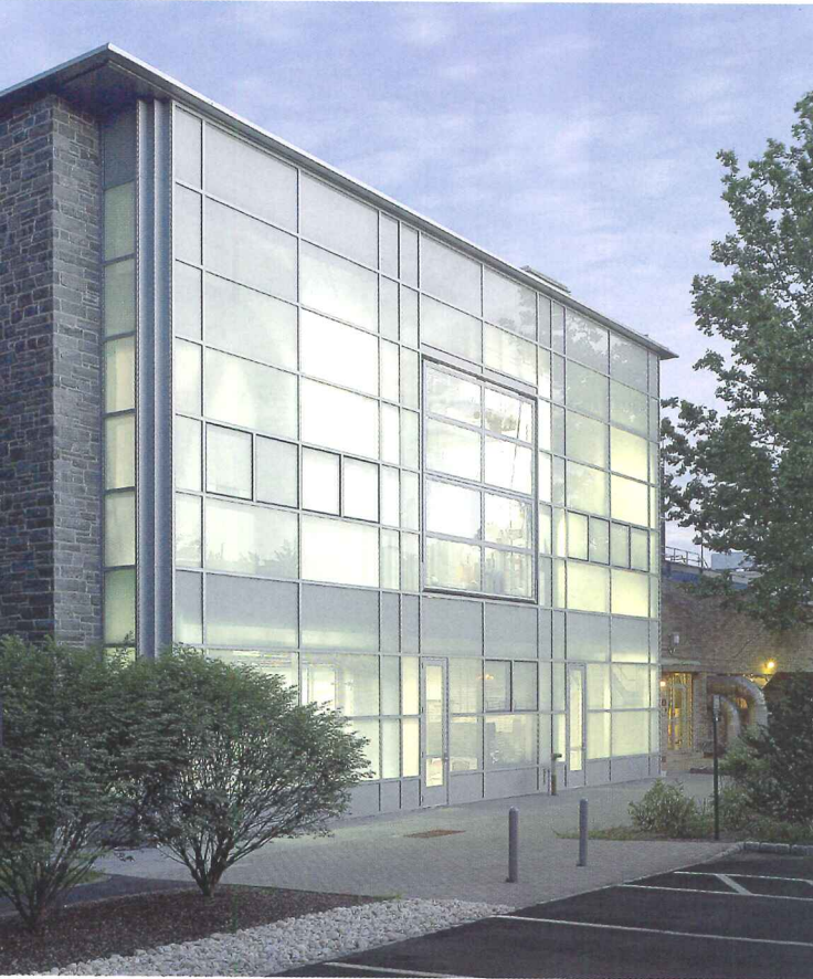
Princeton University Chilled Water Plant expansion, Princeton, N.J., 2005.
