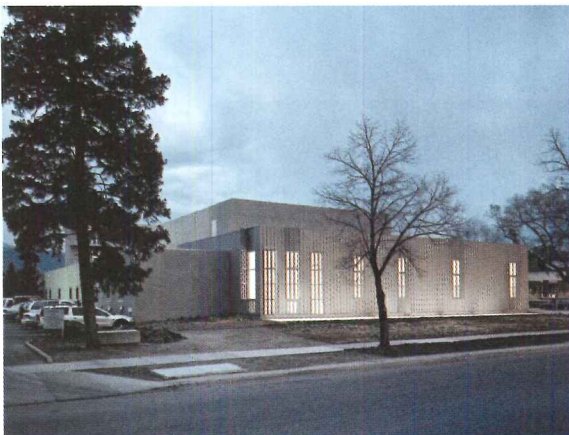
Packard Hall Addition, Colorado College, Colorado Springs, Colorado 2005
