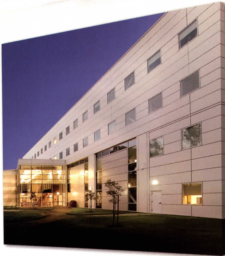
Business & Technology Center California State University V&N Architecture Formawall Dimension Series Insulated Metal Wall Panels FormaBond Metal Composite Wall Panels
