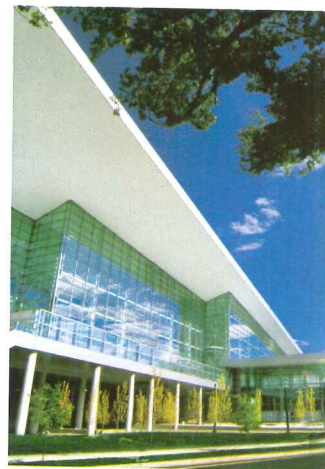
The Colorado Convention Center designed by Fentress Architects. Curtain Wall custom-engineered by Oldcastle Glass®.
