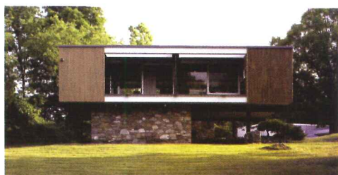
Marcel Breuer's trailer house is going, going ...
