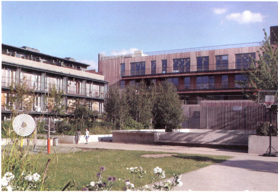
The northern elevation faces a courtyard edged by a housing complex (above left), while a rooftop garden (below) offers stunning views of central London. A concrete stairwell reveals the project's stripped-down aesthetic (above right).
