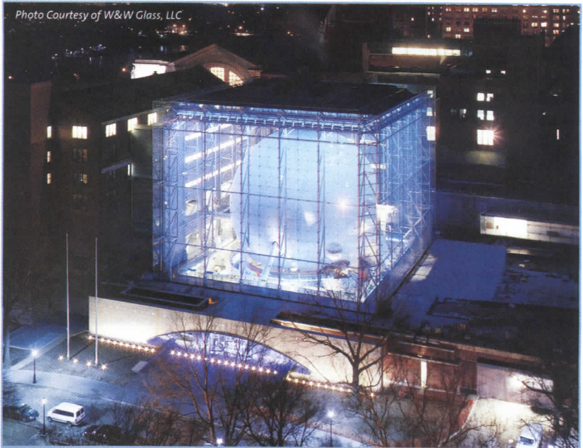
One of the most celebrated and spectacular examples of bolted structural glazing systems in the world is the Rose Center for Earth and Space, American Museum of Natural History, New York City, NY. Architect: Polshek Partnership Architects LLP.
