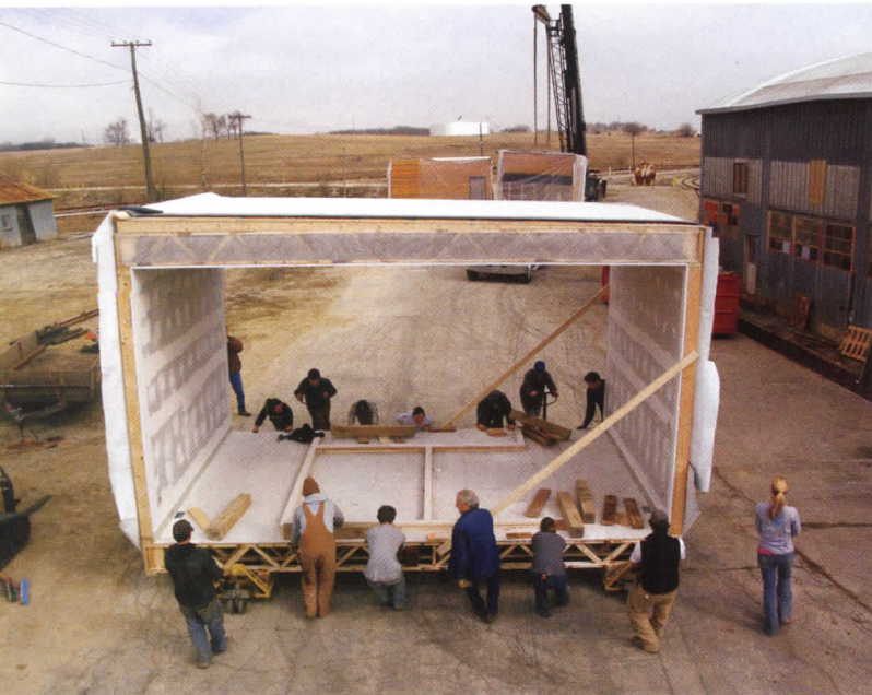
Students prepare to load one of the prefabricated modules of the 5.4.7 Arts Center onto a truck (left); later, it was hoisted into place
