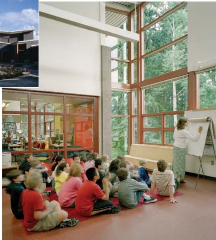
At Benjamin Franklin Elementary School (top), sliding glass doors between classrooms and shared multiuse spaces (above) support the district's teaching philosophy, but compromise the acoustical isolation.
