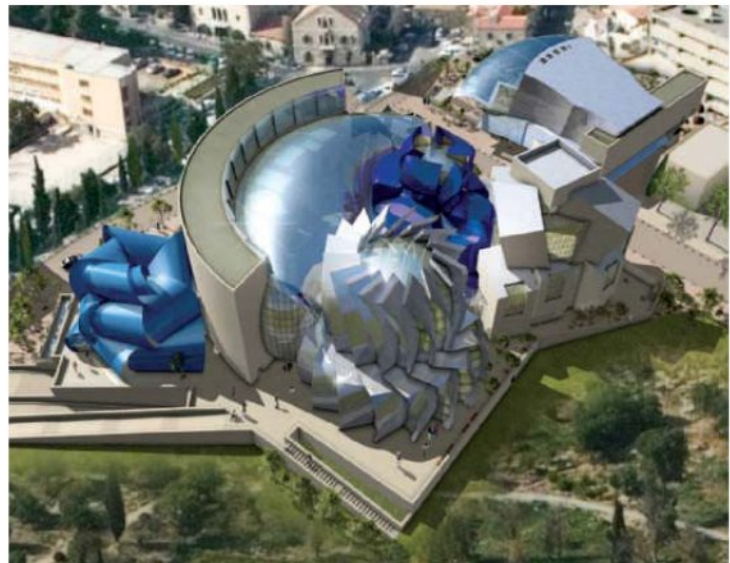
Construction of the Gehry-designed museum was halted three years ago.
