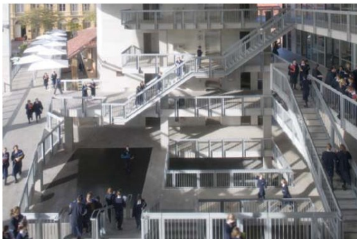
A new creative-arts building at Brisbane Girls Grammar School is organized around a multistory, activity-filled hub.
