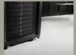
esd flooring systems
