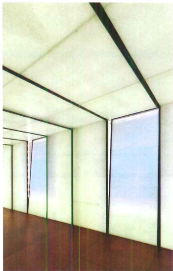
The translucent panels tilt open in front of existing windows (above).
