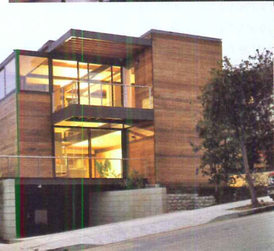
Designed for LivingHomes founder Steve Glenn, this house was built over eight hours on April 13th, 2006, from 11 prefabricated modules – each weighing an average of 10,000 pounds.
