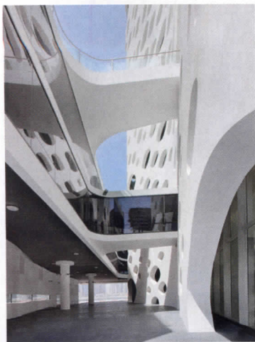
ABOVE: The two-story elevated podium links to the concrete exoskeleton and the glass tower via bridges. The rear is open at the ground level to permit access to the plaza overlooking the bay.
