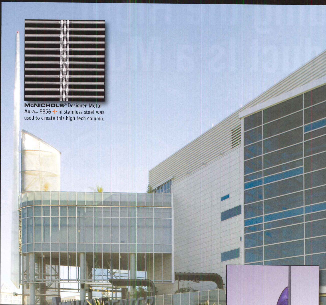
The Amway Center's 180-foot needle tower is a beacon in the city of Orlando. The column is made of McNICHOLS® Designer Metal - Aura™ 8856 + in stainless steel.
