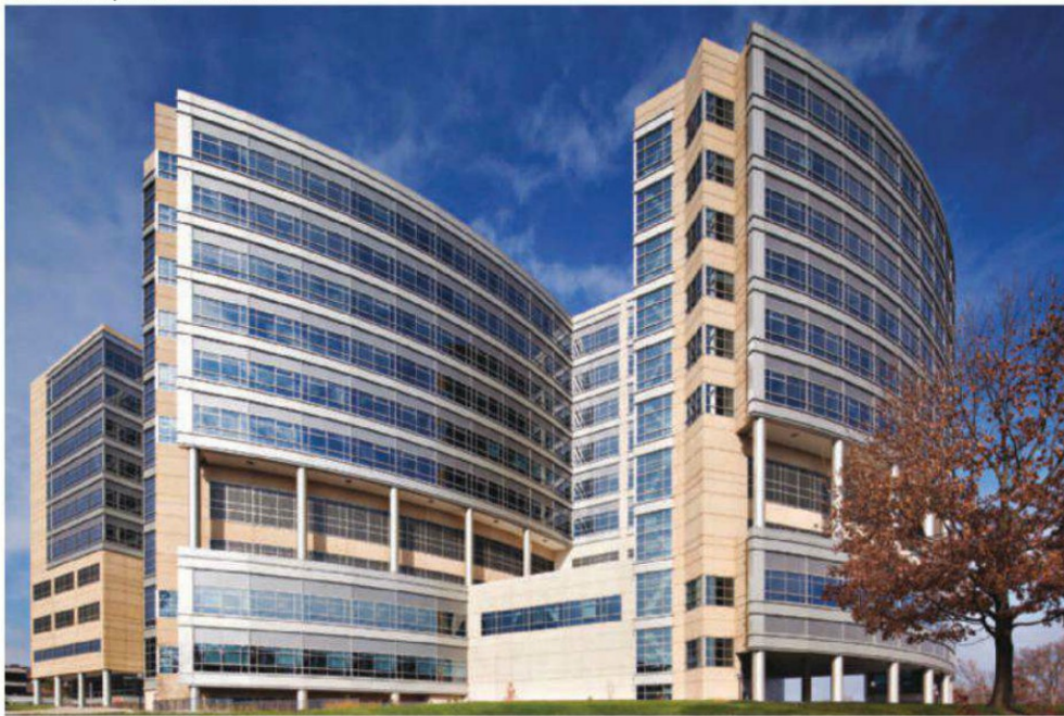
The University of Michigan C.S. Mott Children's Hospital and Von Voigtlander Women's Hospital was designed by the firm HKS to use low-E glazing with low reflectivity and a neutral appearance.
