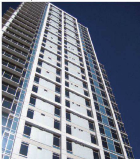
The Sapphire Towers in San Diego have glazed openings with a minimum 45-minute fire rating.
