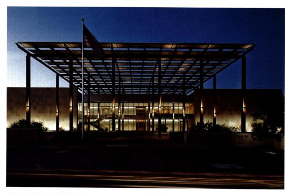
**JOHN M. ROLL U.S. COURTHOUSE** Ehrlich Architects' \$24 million courthouse in Yuma, Arizona, includes photovoltaic panels mounted on a weathered-steel entry canopy that supply 20 percent of the building's electricity.
