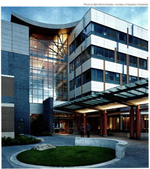
Using targeted glass formulations on different elevations helps optimize light transmission and thermal performance, as at the Swedish Medical Center in Issaquah, Washington, designed by CollinsWoerman Architects.
