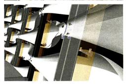
steel columns covered with more delicatelooking steel shrouds evoking traditional Middle Eastern mashrabiya screens. The combination produces a permeable building skin for the 65,000-seat multipurpose facility designed to FIFA soccer guidelines and international track-and-field standards.
