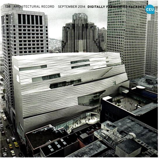
in the U.S. has devised a cost-effective plan to produce over 700 unique panels for what is one of the largest and most significant digitally fabricated building projects to date—the main facade of the San Francisco Museum of Modern Art (SFMOMA) expansion by New York—and Oslo-based Snøhetta.
