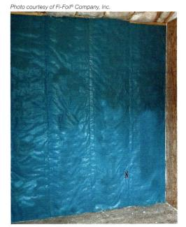
For air sealing of the envelope and to control facade system emittance and radiant heat to improve thermal performance, some projects use hybrid insulation assemblies with enclosed air spaces and low-E reflective insulation.
