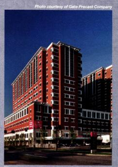
The precast included several different finishes with five colors of thin brick. producing a range of color that is common to the handset-brick and stone used on adjoining buildings.
