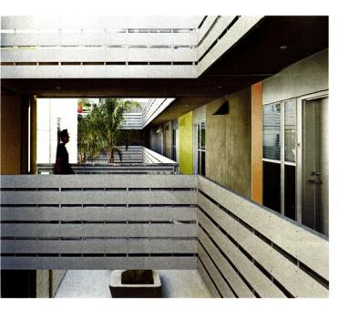
MATERIAL MATTERS Fiber-cement siding, perforated aluminum-zinc coated sheet-steel panels, and integral-pigment stucco are durable and easy to maintain, suiting the complex's modest operating budget.
