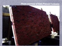
recast panels consist of a 3-inch exterior wythe of concrete, with a 5/8-inch layer of embedded thin brick, a middle 2 inches of insulation with ship-lapped edges, and an interior 4-inch structural wythe. Thin brick can also be returned for edges and corners if desired as seen in this photo.
