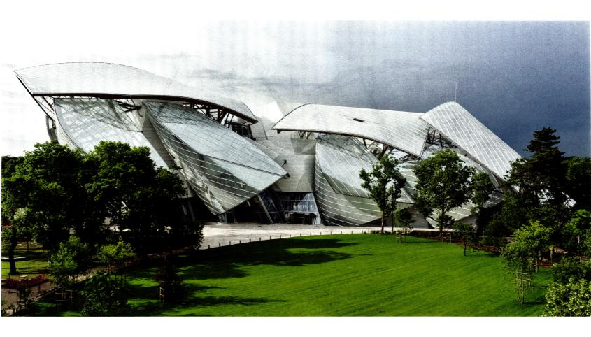
TRIM THE SAILS Anchored in a water feature above the cascade to the east (opposite) or viewed from the Jardin d'Acclimatation to the north (above), the building shows off the elaborate web of steel and wood elements that hold the curving glass canopies aloft. The base of the building. below grade, is French limestone, the same stone used for the lobby floor.
